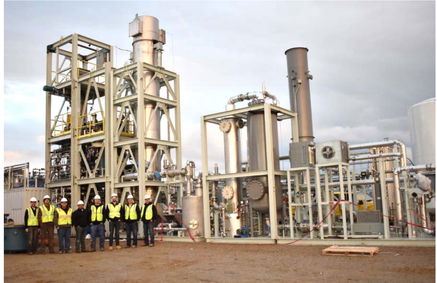
Sierra Energy team at Fort Hunter Liggett Site during commissioning
